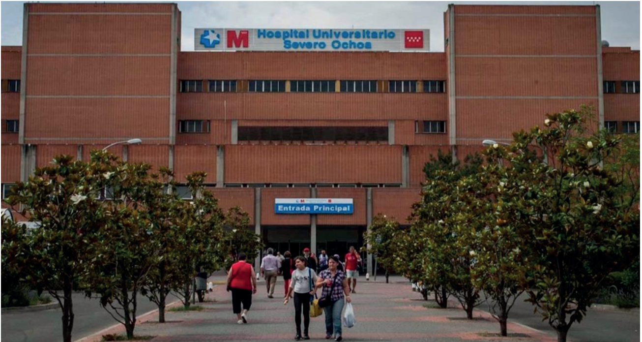
Figure 9. The hospital Severo Ochoa in Madrid.
