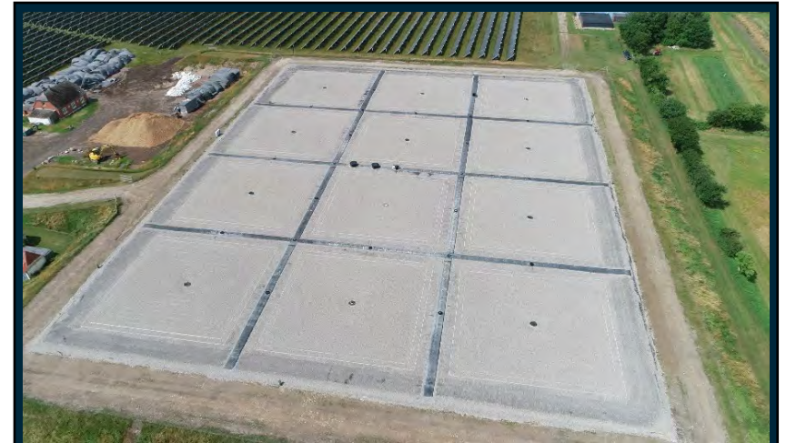
Pit Thermal Energy Storage in Marstal
